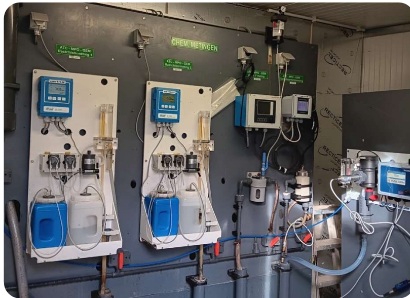
Figure 4– Swan Ami Code-II (2 each) versus Pyxis ST-765SS-FCL Sensor / FR-50 Flow Reservoir / Walchem i6
